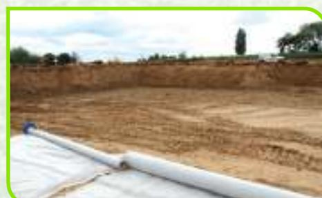
**POUR ENSUITE PROCÉDER À LA STABILISATION DU TERRAIN PAR INJECTION DE CHAUX AINSI QUE PAR LA POSE D'UN FILM GÉOTEXTILE**
